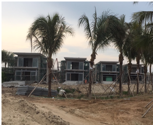
Xây dựng Villas – Construction of Villas
