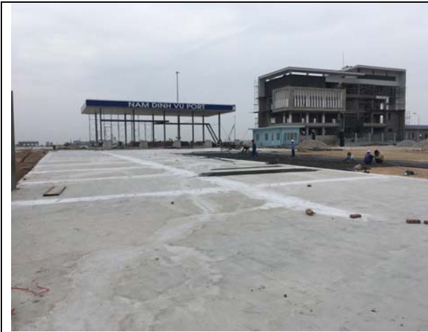
Thi công kho bãi – Construction of yard
